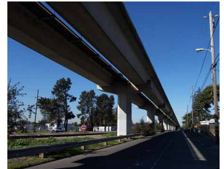
Elevated BART tracks
