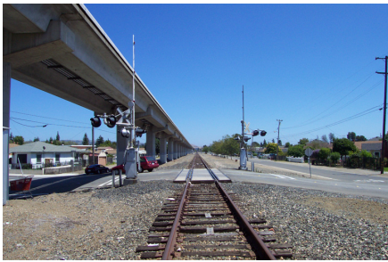
Elevated BART tracks along Western Boulevard
