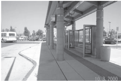
AC Transit Service to the Castro Valley BART station
