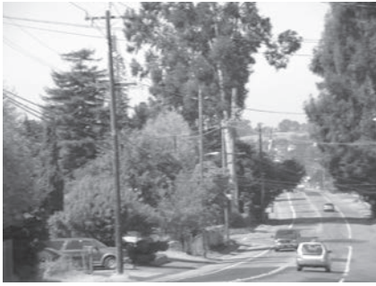
Roadway striping helps to reduce traffic speeds.
