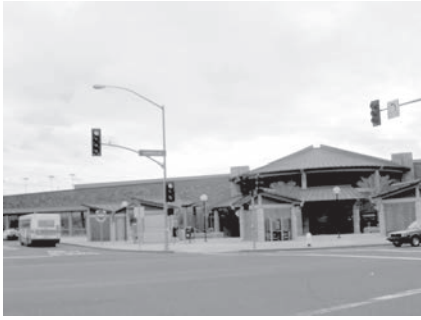
Castro Valley BART station
