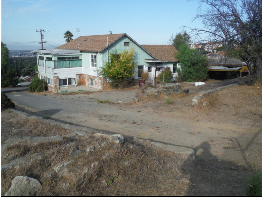
Photo 7: View west of rear of 3289 D Street. Rock retaining walls evident.
