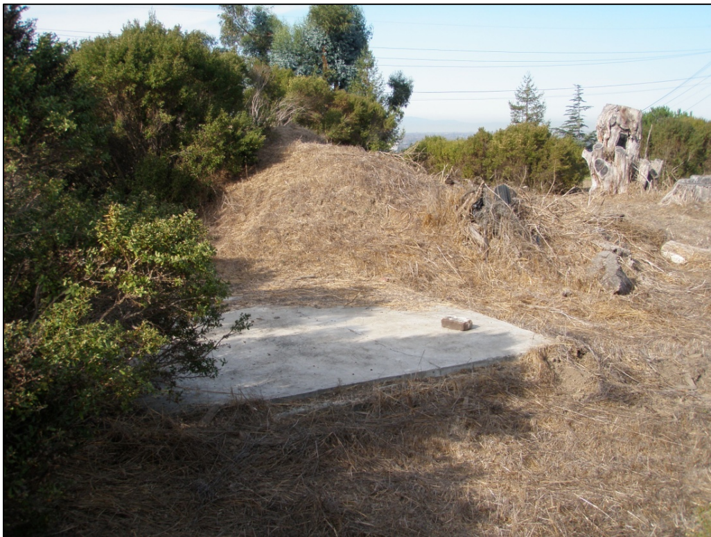
Photo 2: View northwest. The concrete pad and berm at the rear of 3291 D St.
