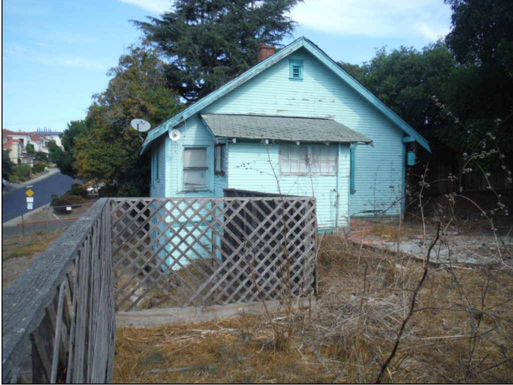
Photo 17. View north of rear of residence at 3247 D Street.
