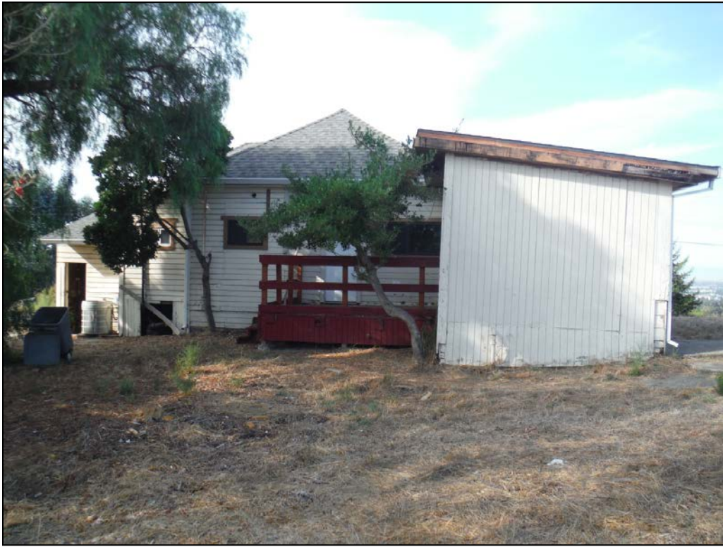
Photo 11. View west of east elevation of 3291 D Street.
