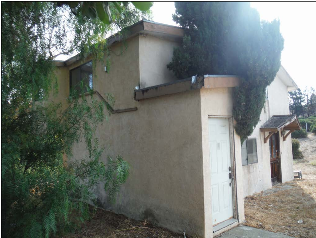
Photo 14. View southeast of renovated garage at 3291 D Street. Enclosed stairway evident.
