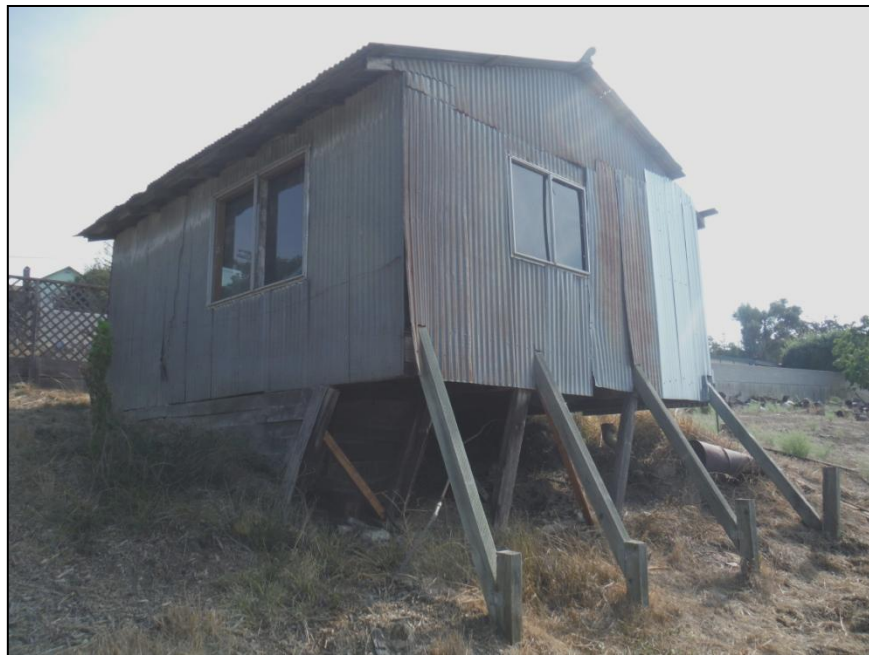
Photo 1. View southeast of shed behind 3247 D Street.
