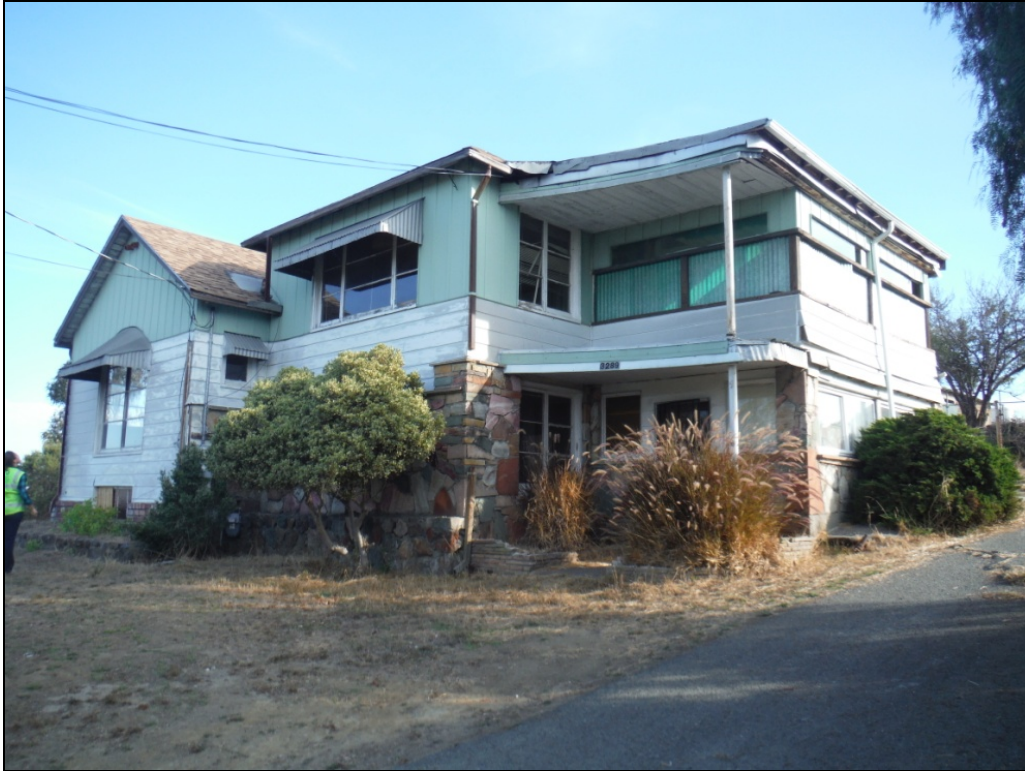
Photo 5: View northeast of facade of 3289 D Street.
