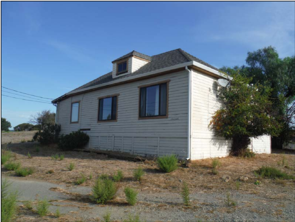
Photo 10: View northeast of west elevation of 3291 D Street.
