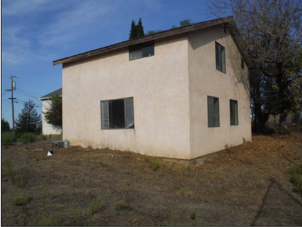
Photo 13. View northwest of renovated garage at 3291 D Street.
