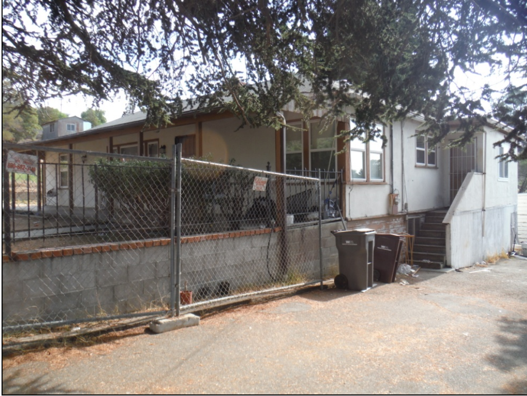
Photo 19. View southeast of facade of 3231 D Street.
