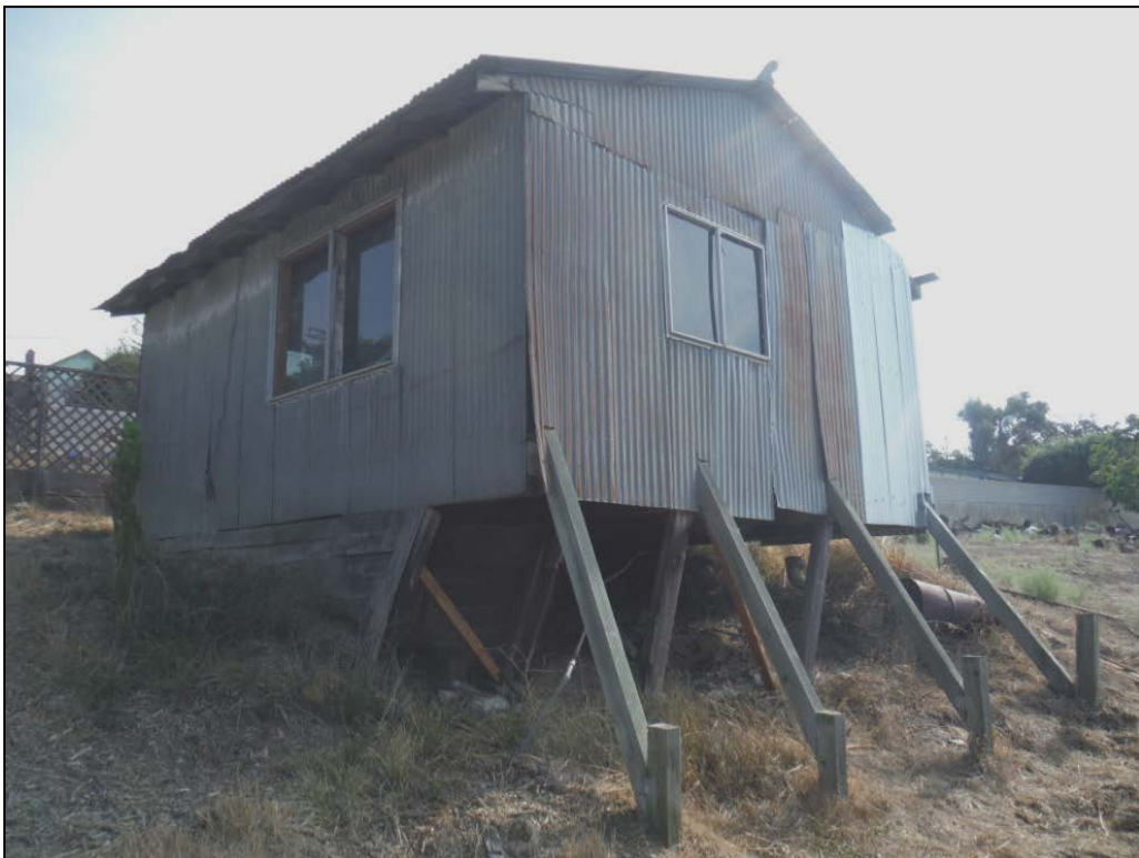
Photo 18. View southeast of shed behind 3247 D Street.
