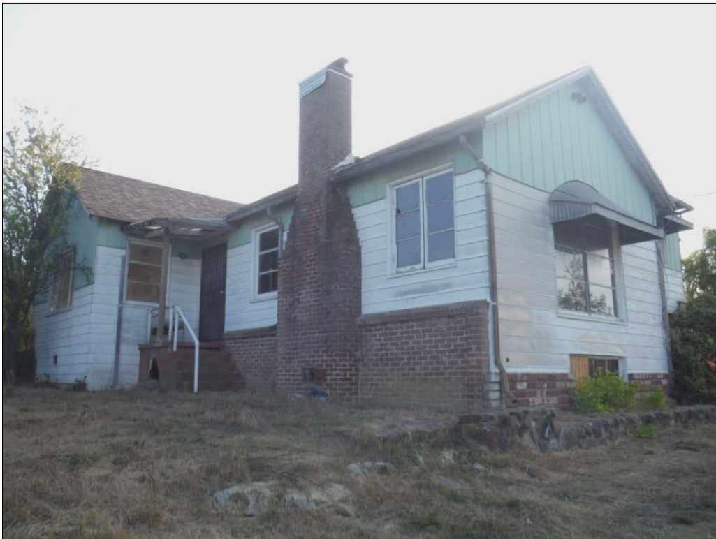
Photo 6: View southeast of facade of 3289 D Street.
