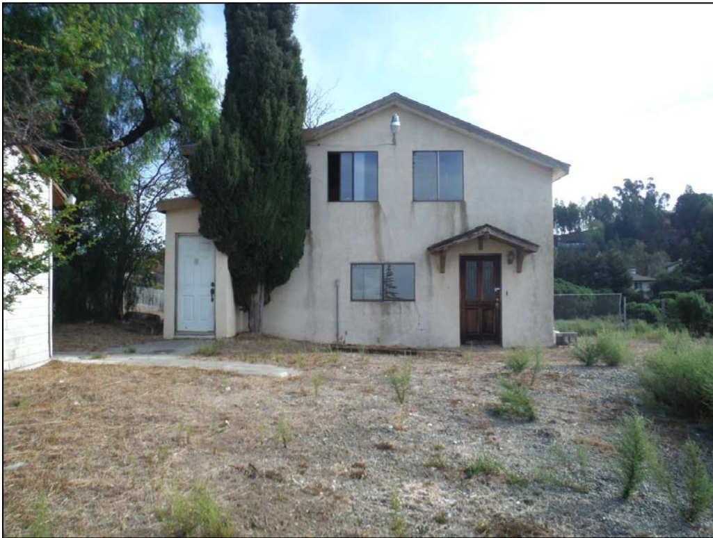
Photo 12. View east of facade of renovated garage (now a residence) at 3291 D Street.
