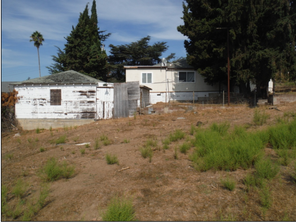
Photo 21. View north of back of garage and residence at 3231 D Street.
