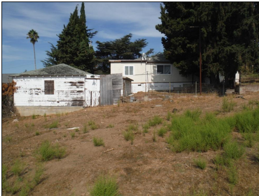
Photo 1. View north of back of garage and residence at 3231 D Street.
