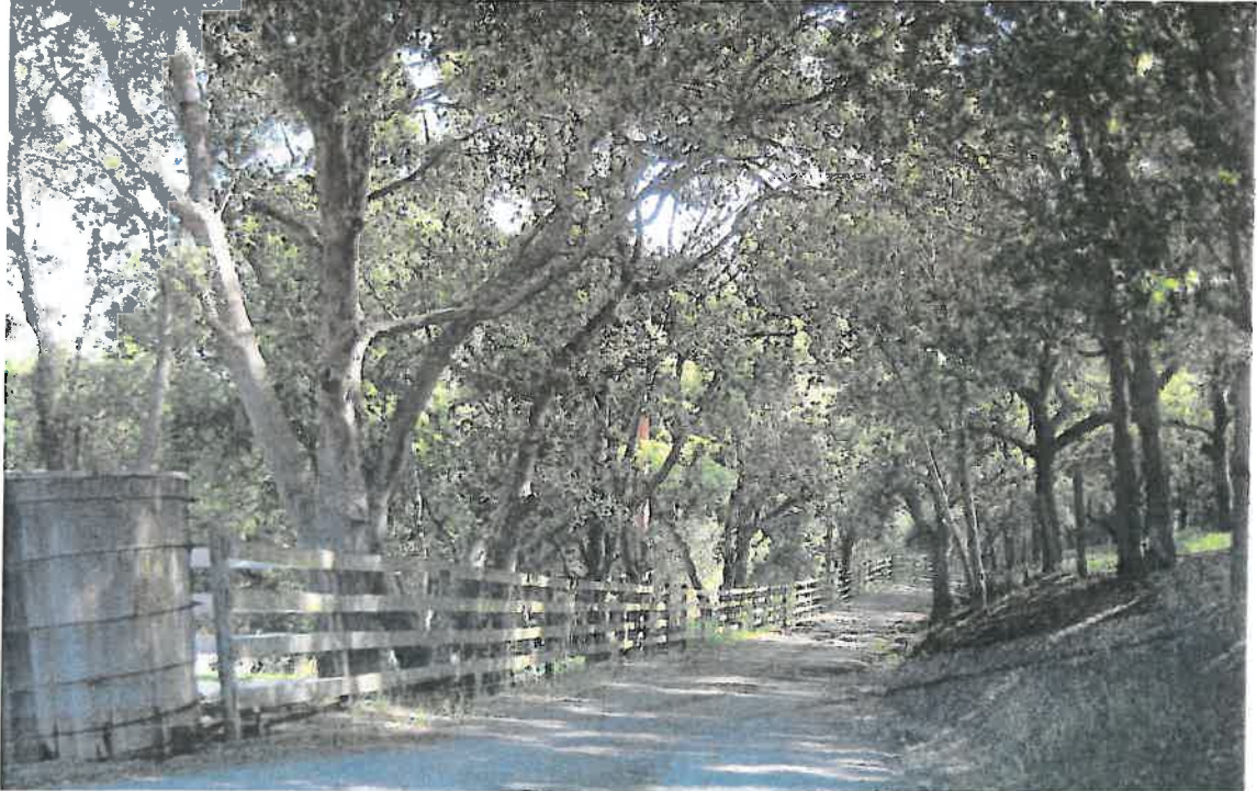
Figure 4 – Typical view of roadway
