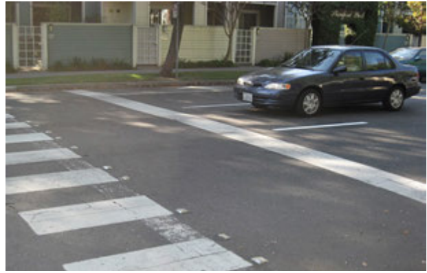
Example of Advanced Stop Bars. At a Signalized Intersection, the Bicyclist will Stop Ahead of Vehicles. Advanced stop bars allow for safer stopping and Starting While on a Bicycle, and Keep the Bicyclist Within Sight for all Auto Drivers.
