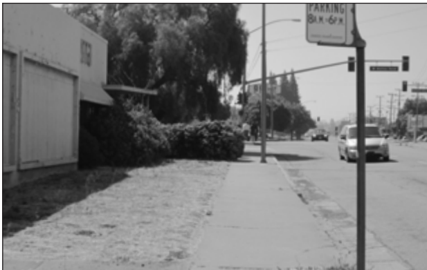
Current Sidewalk Conditions in ACBD West Eden Corridor
