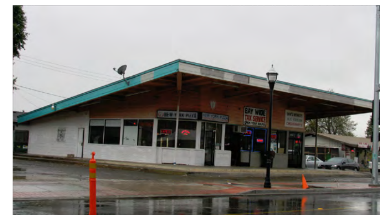
Disinvestment in Structures along East Lewelling Boulevard
