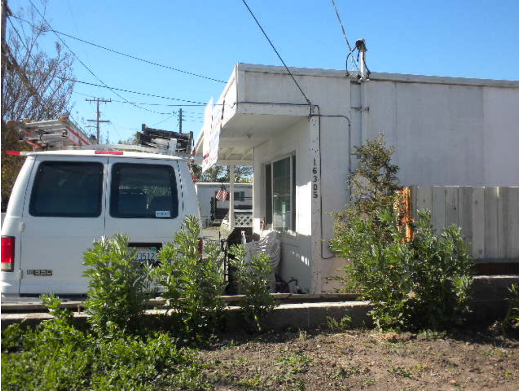
Photo 5: Northeastern Façade of 16305 Kent Avenue Residence
