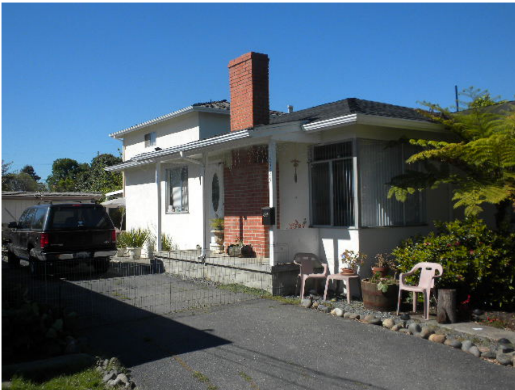
Photo 2: Northeastern Façade of 16325 Kent Avenue Residence
