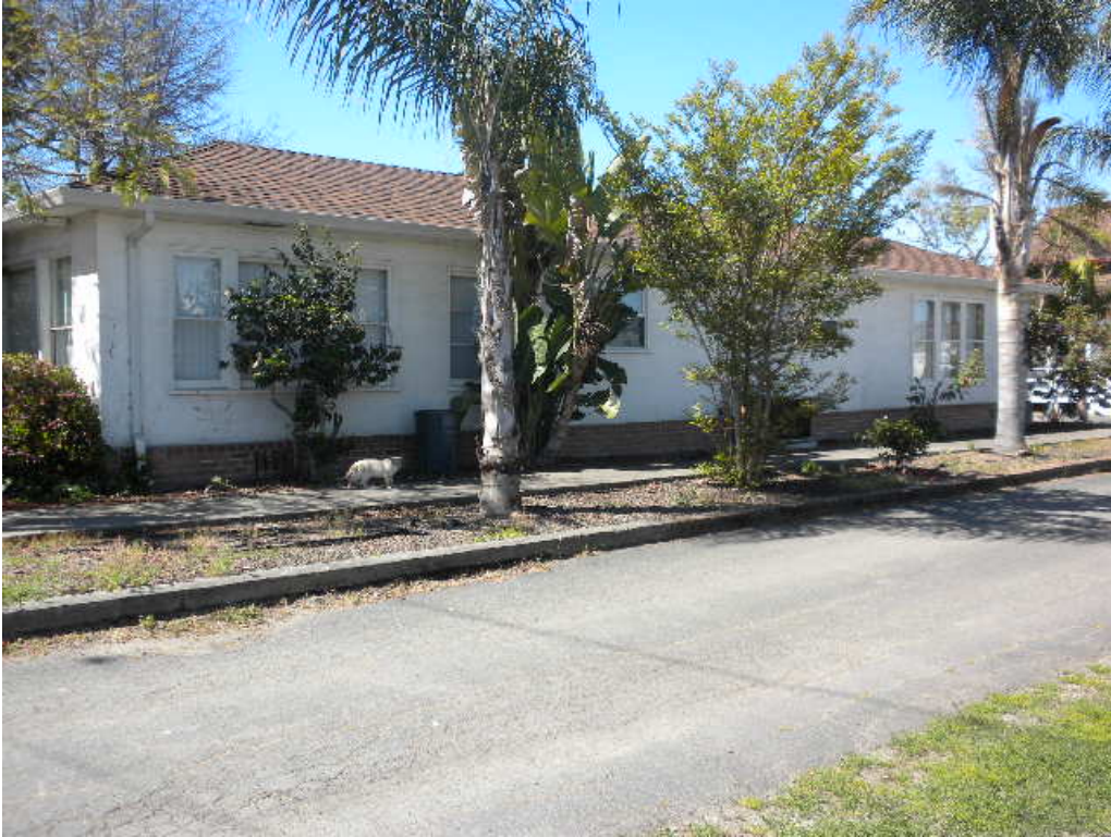
Photo 3: Eastern Façade of 16331 Kent Avenue Residence
