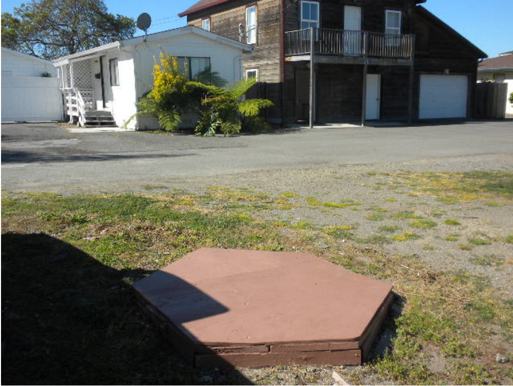
Photo 7: Cistern Access Cover
