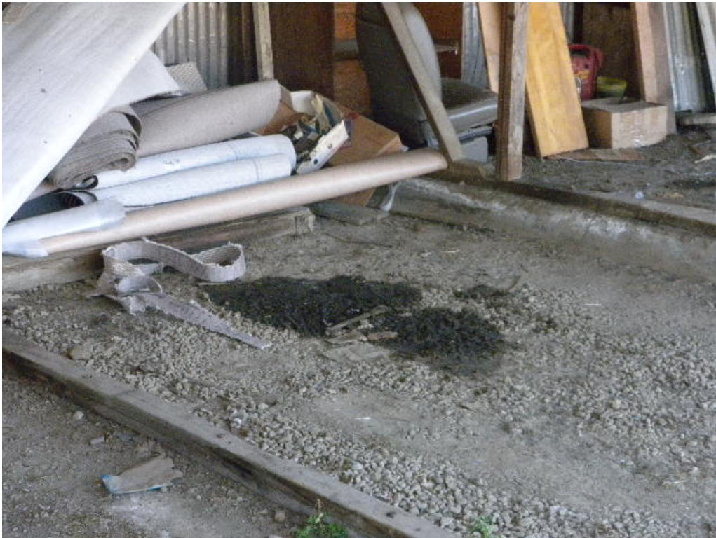
Photo 15: Vehicle-Related Oil Stain in Carport
