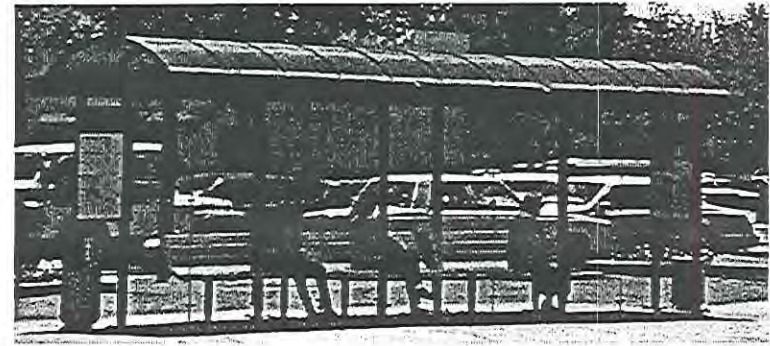
Bus Shelter Daytech
