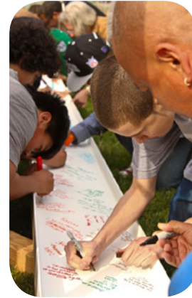
Local youth and community members write positive messages on a 30-foot steel beam erected at the Ashland Youth Center site in April.
