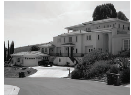
Develop new height limits and new methodology for calculating height appropriate for hillside lots.
