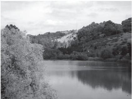
Cull Canyon Lake is a distinctive component of Castro Valley's visual identity as well as a flood control facility.
