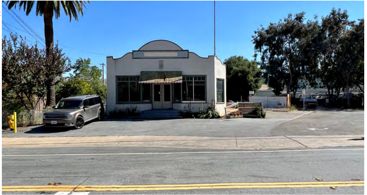
Looking South at vacant commercial building
