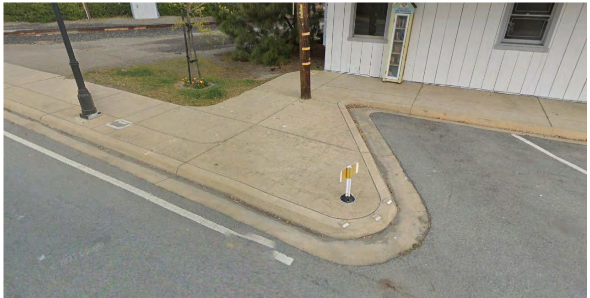
Looking Northwest at existing Area 6 sidewalk
