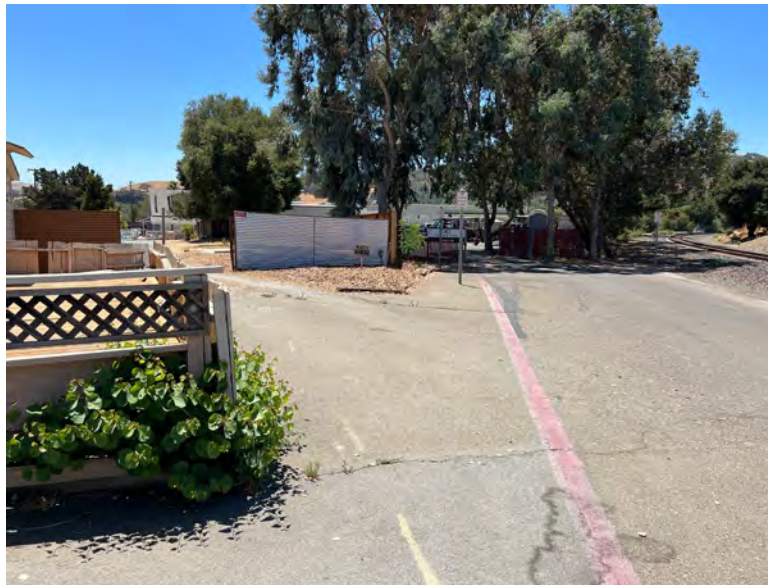
Looking South at outdated striping adjacent to vacant commercial building
