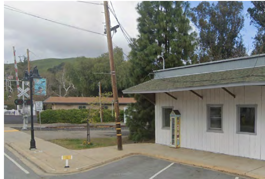
Looking Northwest at existing Area 6 sidewalk
