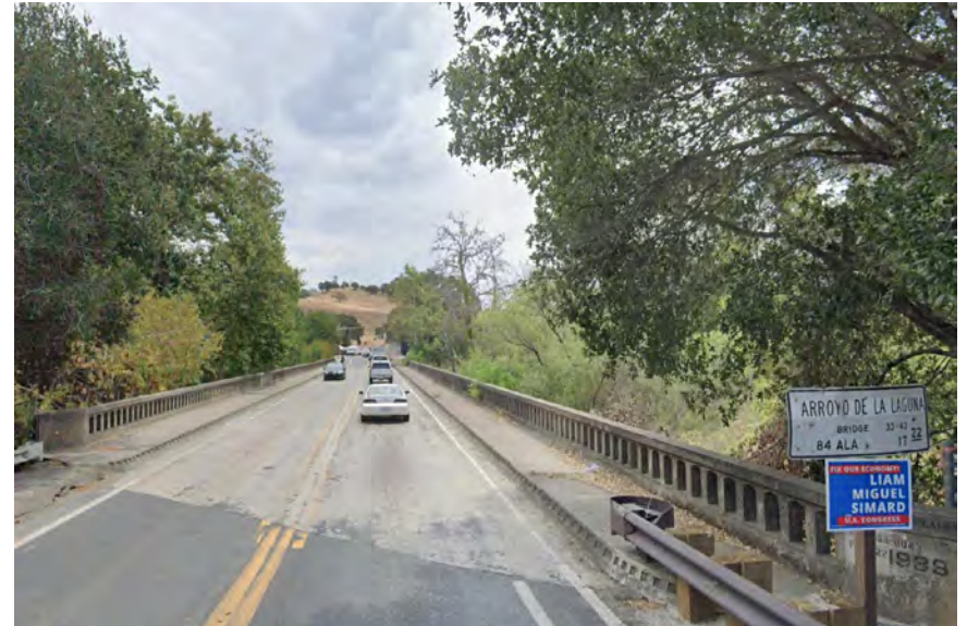
Looking East across the bridge
