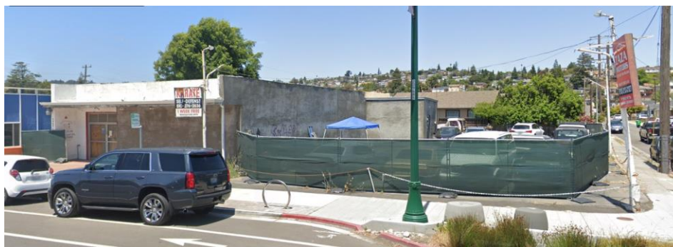
Figure B-2. The most recent Google imagery of 17144 and 17156 E 14 TH (June 2023).
