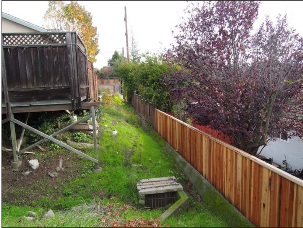
Photograph 5 - Storm drain inlet and easement at southeast corner of Project Site
