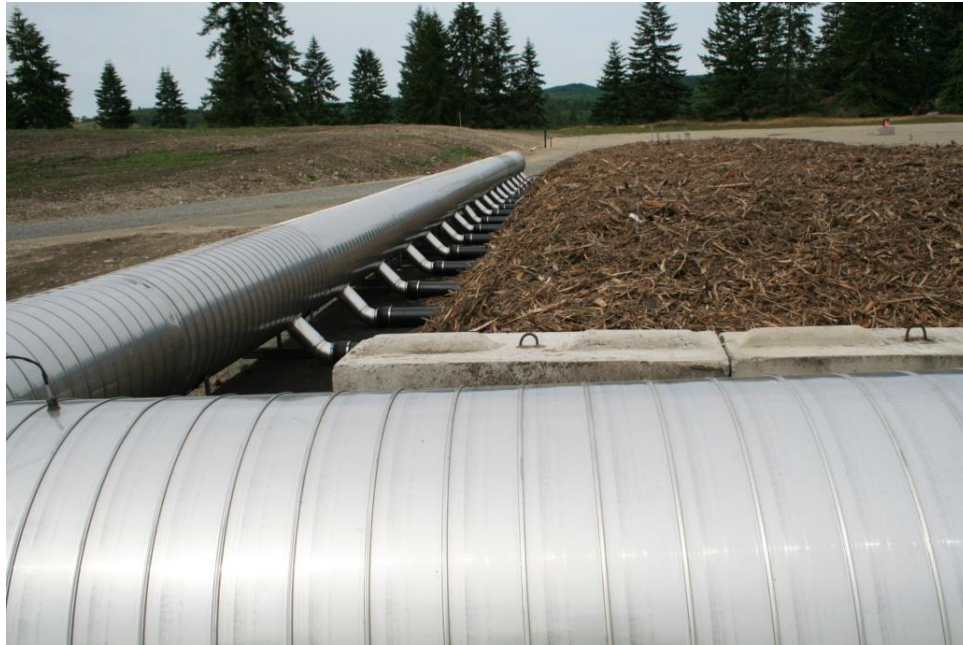
Figure 4 Aerated Static Pile Biofilter
